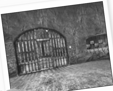
... but 2nd chamber's gate closed when 1st chamber's opened.
