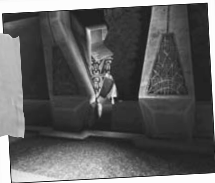
Crack in wall led into Beetle Cages.
