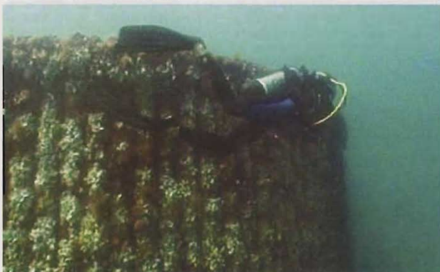
A sea water intake. A desalination plant can suck up to 20 million litres per hour but the design of the intakes ensures that the flow into the intake is mild enough to have little effect on marine life (including divers!).
