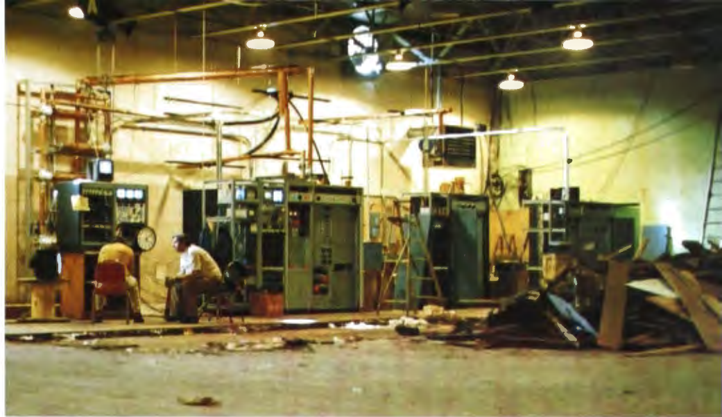
The major effort was in getting the TV station on-air for the 1977 baseball World Series. Even amid the debris of converting the sports arena into a broadcasting station, the TV transmitting system aired the first game. At left is the makeshift "master control" with the oversize clock.
