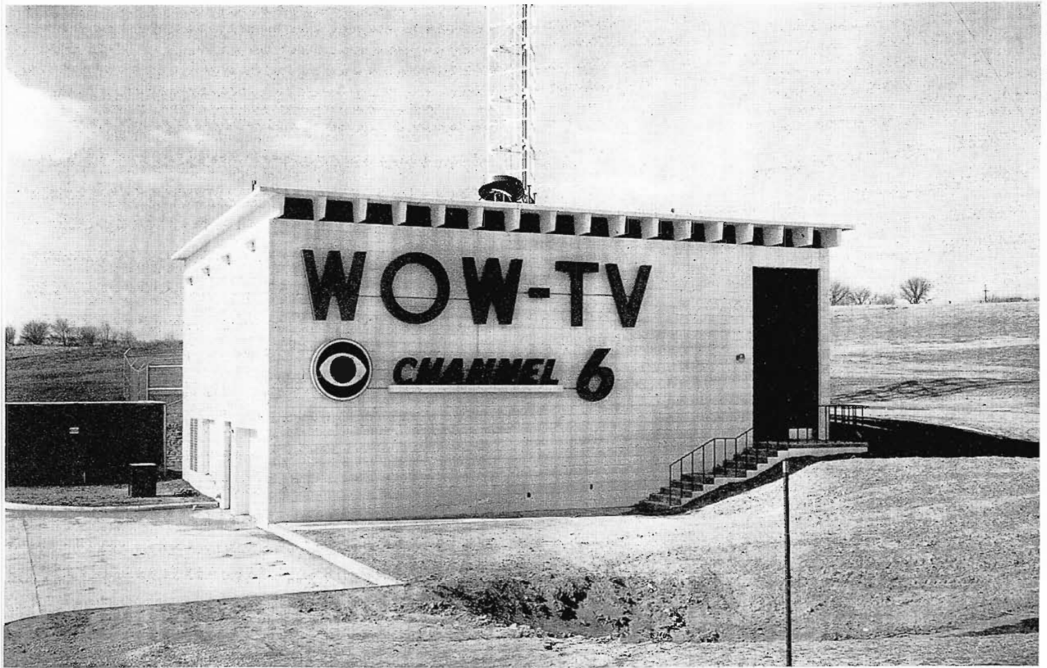
FIG. 2. This is the new WOW-TV transmitter building and tower completed in November, 1966 and houses the RCA TT25-EL VHF Transmitter. It's on a "tower farm" at 72nd and Crown Point outside of Omaha. Located at this same location are two other new towers for stations KMTV and KETV.
