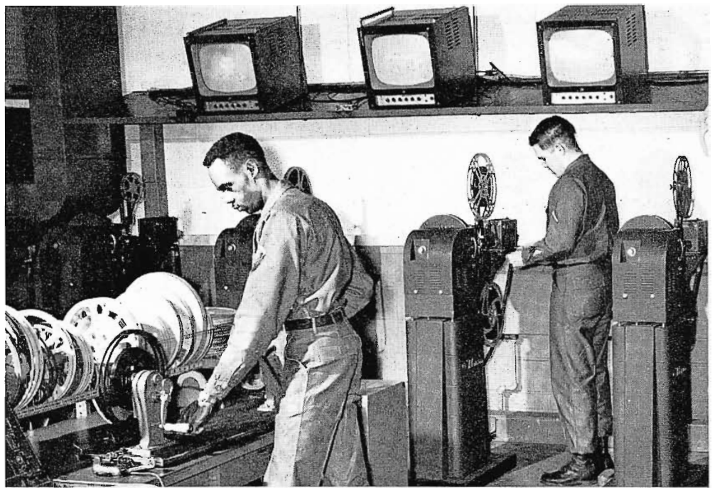
FIG. 4. Nine TV film chains are used to distribute training films to classrooms.
