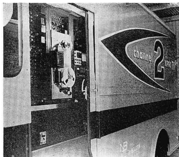
KPRC-TV, Houston, Mobile Unit features permanently-installed RCA TRT-2 Recorder for compatible quadruplex TV Tape recording in the field.
