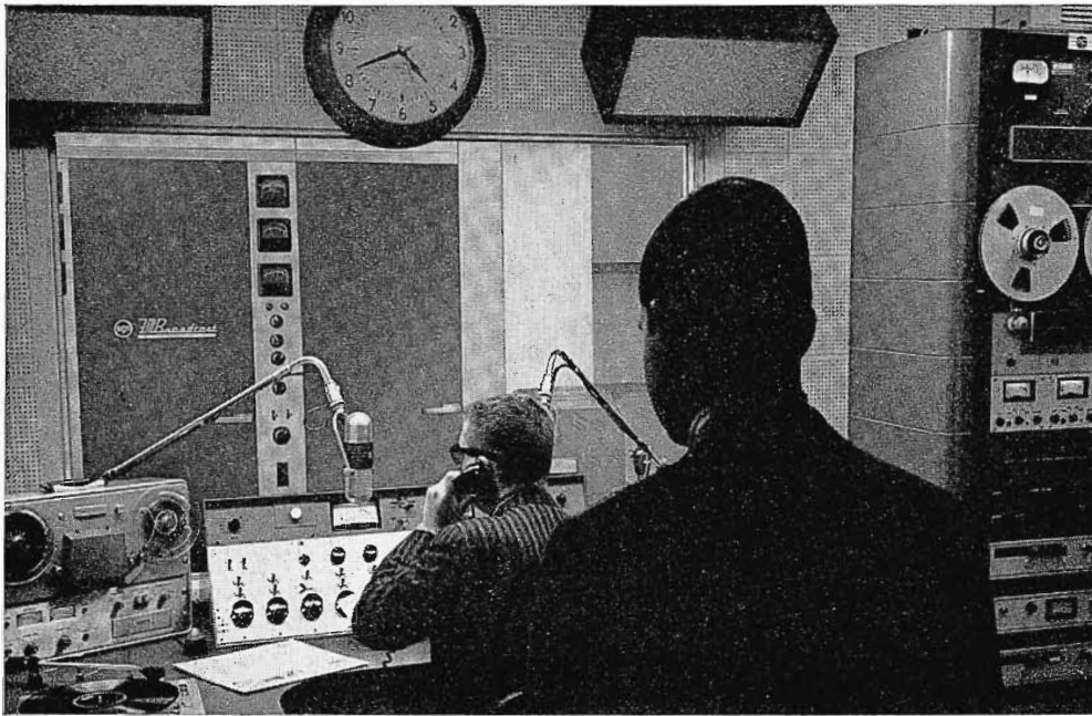
FIG. 1. KRAV Studio A control. Announcer Robert Thomas takes a phone call from a listener. The picture window immediately beyond the BC-7 control console allows almost continual monitoring of the BTF-5D transmitter meters. Mikes are 77-DX velocities.
