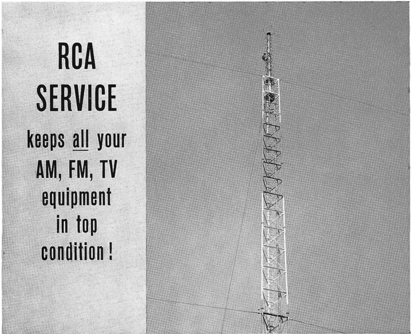
Antenna System Measurements
