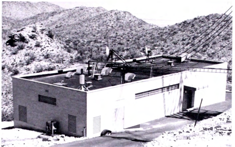
FIG. 3. Exterior view of transmitter building atop South Mountain looking north toward the Coolidge-Casa Grande Valley. Two microwave dishes on the roof link with the KPHO studios, and one can be used for remotes. Transmission line is run from the top of the building to the tower.
