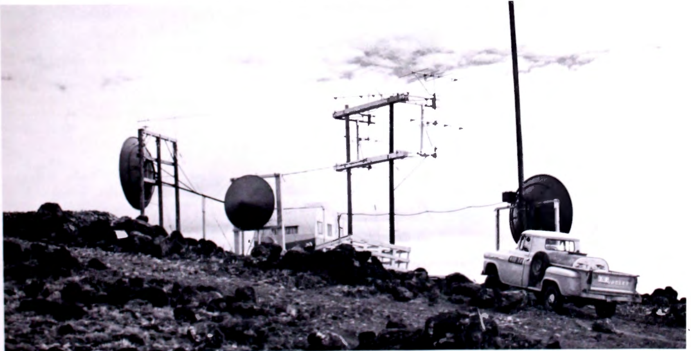
FIG. 3. Receiving location at Albion, Idaho. Parabola at the right faces Coon Peak, 136 miles distant. Parabola at the left faces East Butte, 89 miles away.
