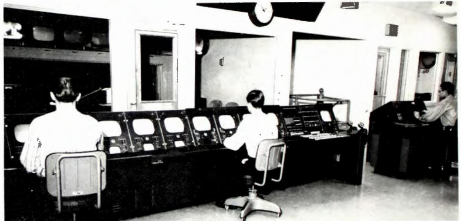
FIG. 14. TV Master Control. At left, Paul Wilson and George Alsobrook are at the video controls. At right, Mac Hix is at master audio console. Sub-control A is in front of video console. Master panel for TS-40 Switching System is at right end of video console.
