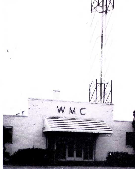
FIG. 8. Transmitter building is located eight miles from studio. Main and auxiliary towers are shown.
