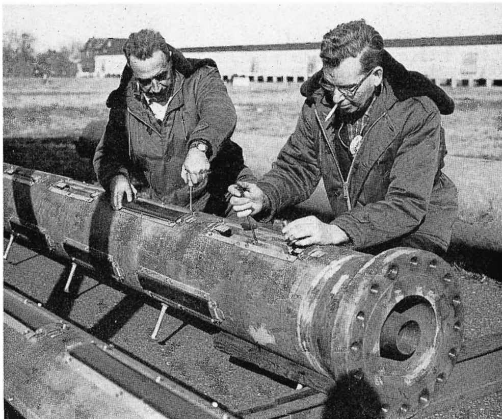
FIG. 2. Tuning plates and slot covers are attached before the TW antenna undergoes fine tuning. Note the hollow inner conductor which is used to run lightning protector and beacon cables to tower base.
