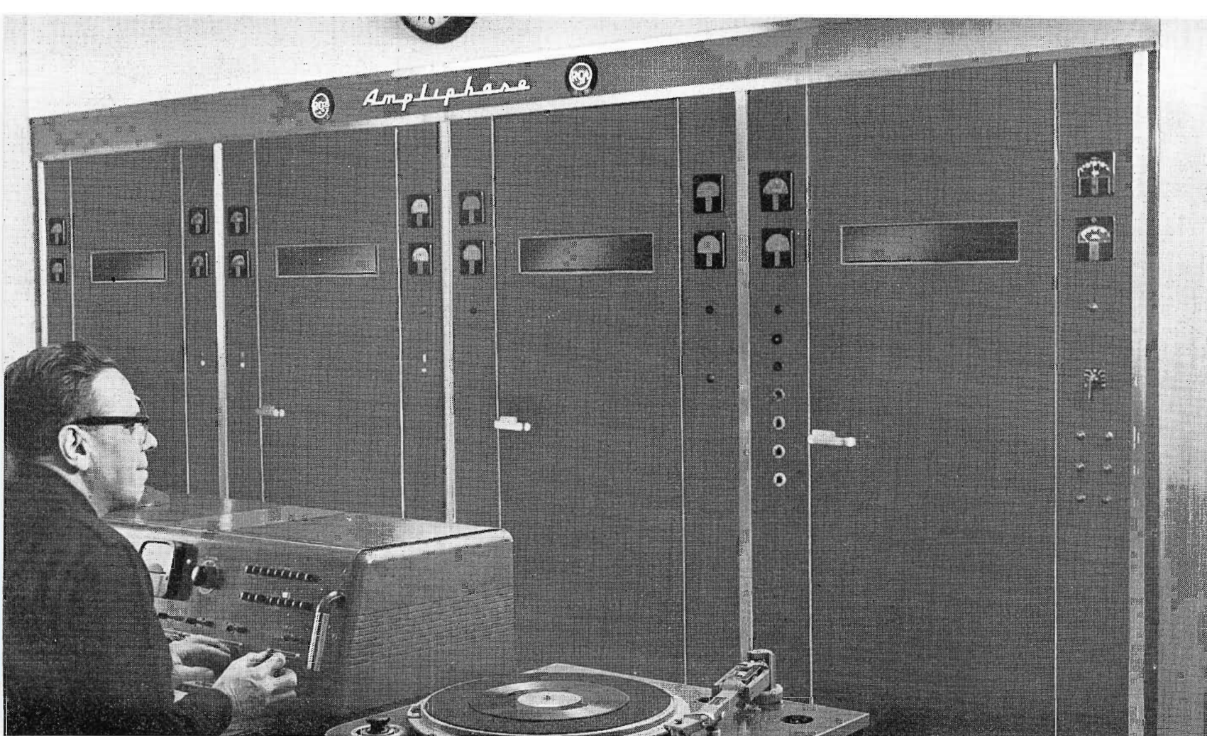
RCA Type BTA-50G transmitter at the WINS transmitter building in Lyndhurst, New Jersey, showing Al Jorgenson at Console.
