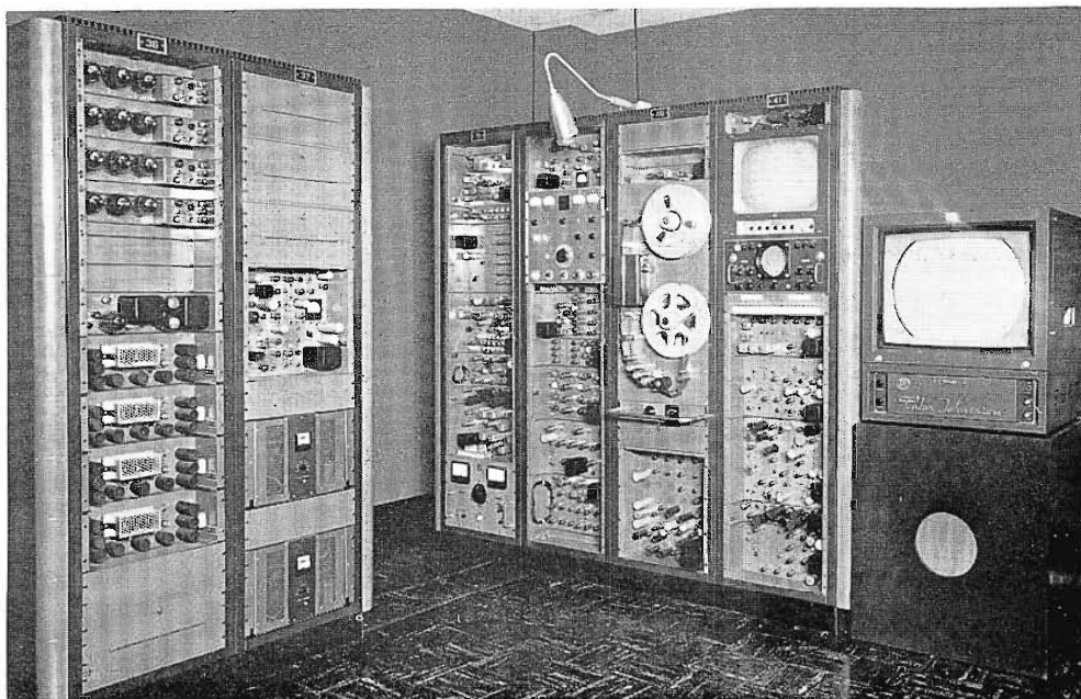
FIG. 4. The RCA Color Video Tape Recorder is shown in a corner of the WBTV telecine room. This area was reserved for video tape as a part of the station's plans for full color operation.
