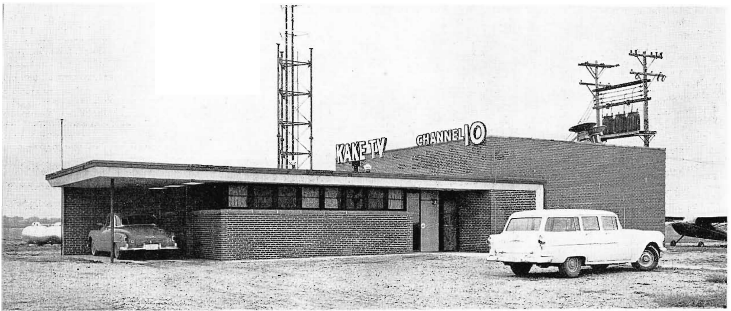
FIG. 23. KAKE-TV transmitter building (includes apartment of resident engineer).
