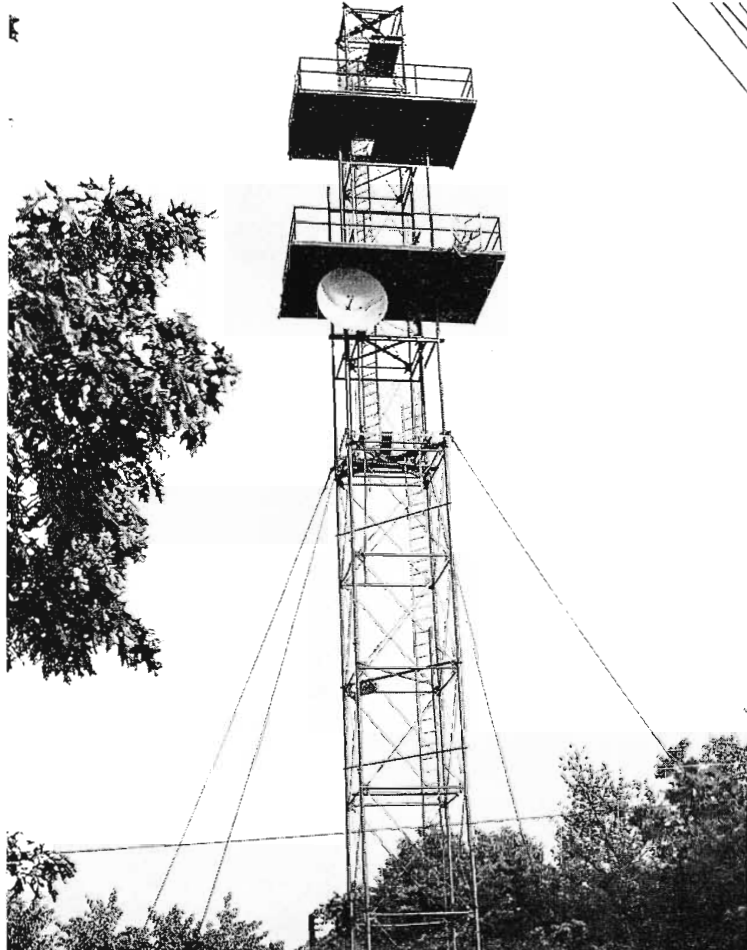
FIG. 8. This transmitting tower at Union Mills, located 2.4 miles from the turntables, emits the test signals.
