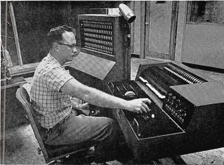
FIG. 9. Lighting control panel located in control room.
