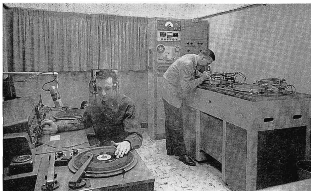
FIG. 22. Control room No. 2 for KAKE radio. Seated at controls is David Dunn. Standing is Radio Chief Engineer, Gene Courtney.
