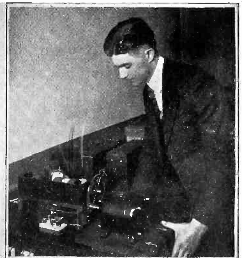
DR. E. F. W. ALEXANDERSON (AT LEFT), INVENTOR OF THE RADIO STILL PICTURE TRANSMITTER, WITH HIS HOME RECEIVER. THE CASE HAS BEEN OPENED AND THE SENSITIVE PAPER IS SEEN ON THE DRUM. THE AMPLIFIER IS BEHIND THE RECEIVER. THE RADIO PICTURE TRANSMITTER, OPERATED BY E. C. BALLENTINE, ASSISTANT TO DR. ALEXANDERSON, IS SHOWN AT THE RIGHT.
