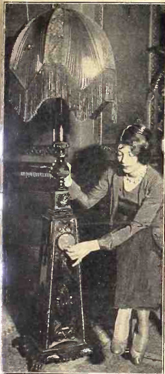
MISS HILLY GRUNBERG turned on a powerful 5-tube radio receiver, installed in the base of a lamp. The dial turns a special type of multiple condenser. The loud speaker is located in the shade. (Underwood & Underwood)
