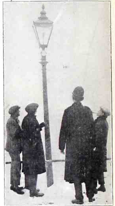
AN electric light or arc lamp in Essex, England, picks up the programs from 2LO and reproduces them with full volume. Engineers claim that the arc lamp acts as a detector, the elements as magnets and the glass as a diaphragm. Policemen, during the lonely hours of the night, gather around this post, to be entertained. (Wide World.)
