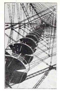
A GLIMPSE of the winding stair-way of the radio tower of "Konigs-wusterhausener." This new tower is 656 feet high, the highest in Germany, and in the world it is second only to the Eiffel Tower in Paris. An innovation will be an elevator within its girders, plans for which have heen completed. (Kadel & Herbert.)
