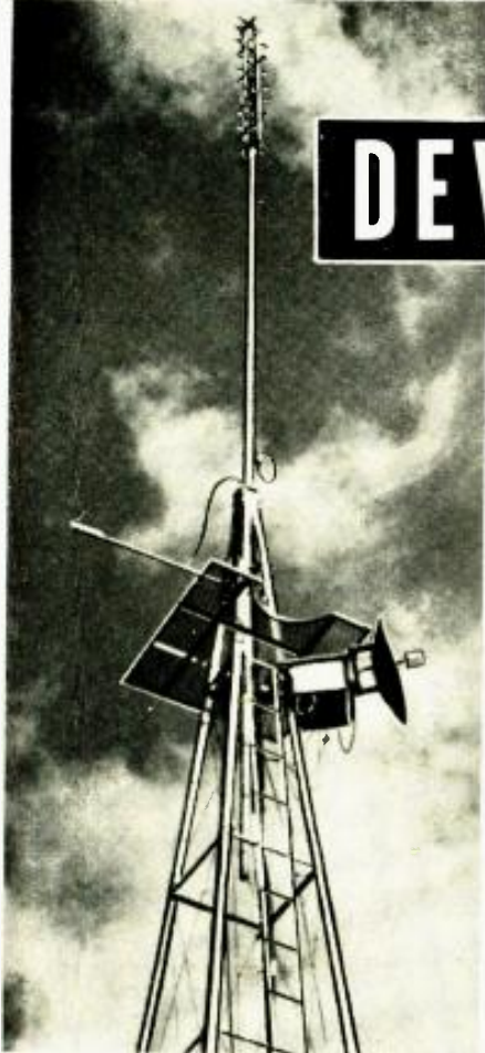
Receiving microwave dish antenna and high-gain channel 82 retransmitting antenna shown on a u.h.f. satellite station tower.
