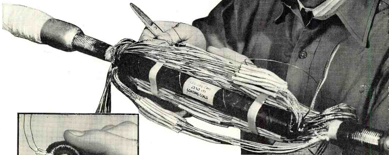
Twenty of the Bell System's newest small loading coils—like the one at the left—are housed in the long black case, mounted in a cable splice. This type of installation permits the economical extension of city cables to serve out-of-town subscribers.
