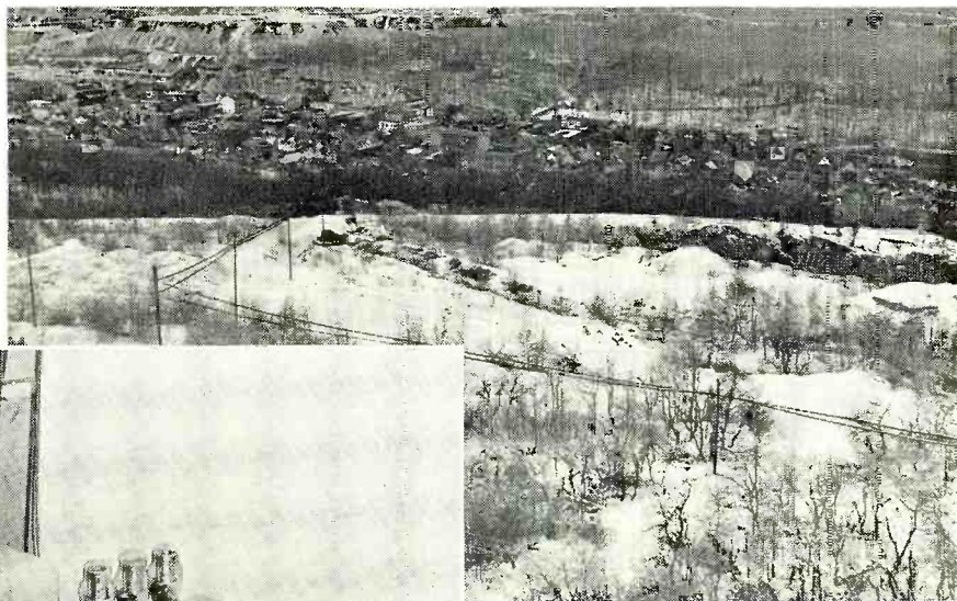
Fig. 5. A view of Panther Valley from Summit Hill. In the foreground are the poles of the Pennsylvania Power & Light Co. which are used to carry the television cables into Lansford. Prior to the installation of the "community aerial," the surrounding ridges of the Blue Mountains cut off the effective reception of video signals.
