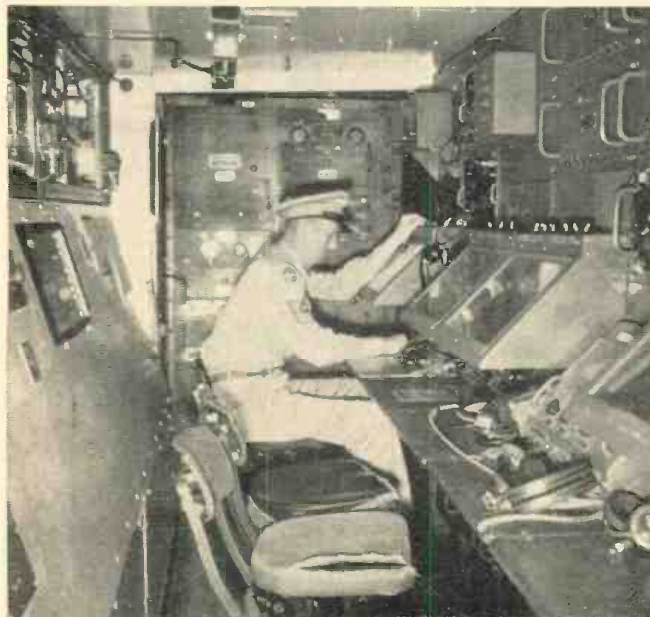
Interior view of the Ground Controlled Approach equipment.
