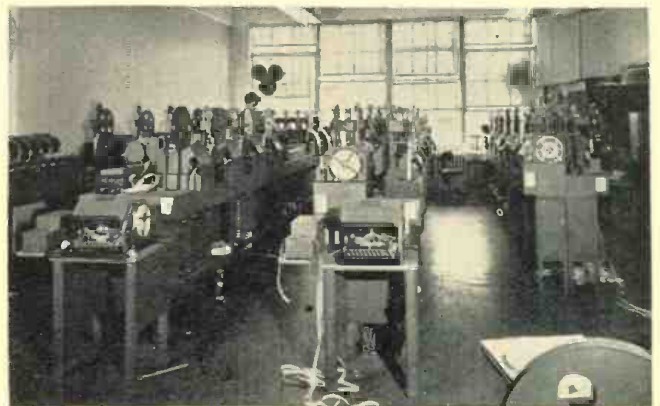
Monitoring equipment, installed at Navy Radio in Washington, D. C., makes a record of all transmissions over the system.
