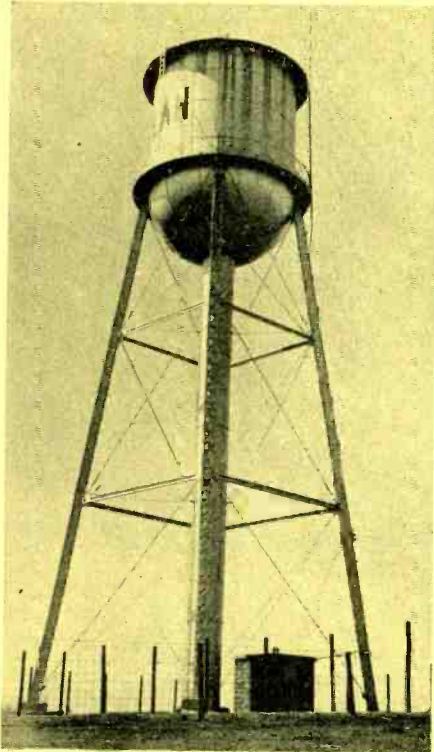
↓ Antenna, atop a water tower, is fed by coaxial cable from the central station transmitter at the base.
