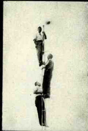
RUGGED! Three "huskies" (total weight over 540 pounds) are easily supported by this steel tower even though no guy wires have been erected.
