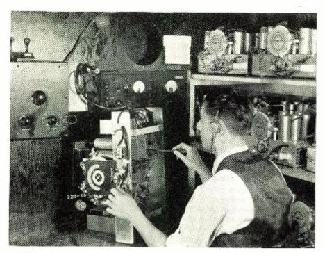
Technician shown adjusting the series padder for correct osc.-preselector tracking.
