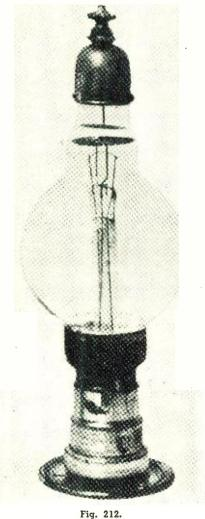
use of cold-cathode tubes and succeeded in making some which operated satisfactorily in wireless work.<sup>294</sup> These tubes were not as sensitive as those of the hot-cathode type although they did possess some advantages. No filament heating battery was required, and their action was not sensitive to small changes in the internal pressure.
