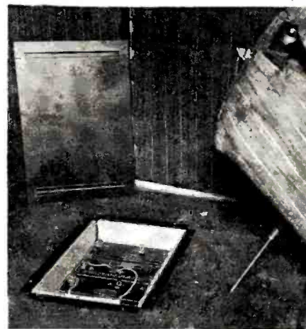
Above is the complete Bosch equipment, which includes "B" batteries and battery box, shelf, tubes, the set and speaker and the tuning control at the lower right with its flexible shaft to receiver
