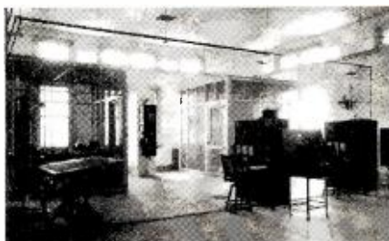
View of monitoring equipment, showing highly sensitive and selective receiving apparatus
