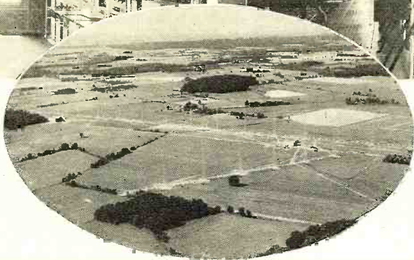
General view of the Bell Telephone transmitting towers at Lawrenceville, N. J. (Courtesy Fairchild Aerial Surveys, Inc., N. Y.)
