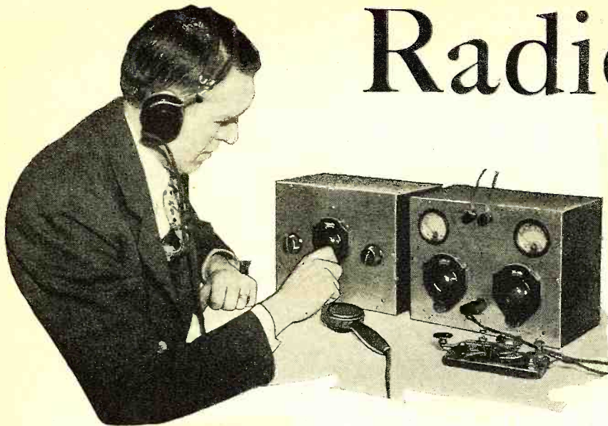
The receiver and transmitter set up for operation
