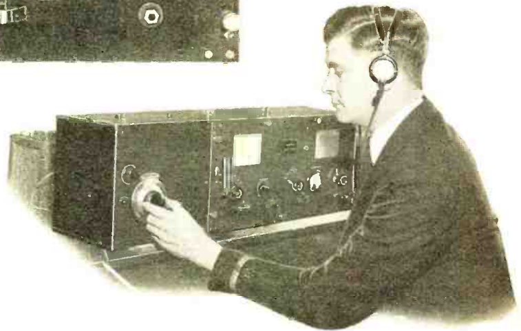
Fig. 4. So that the entire receiver may be readily removed from its metal cabinet, a system of plugs and jacks, as shown at the left, are provided. Above, Mr. Marshall at the controls of his receiver
