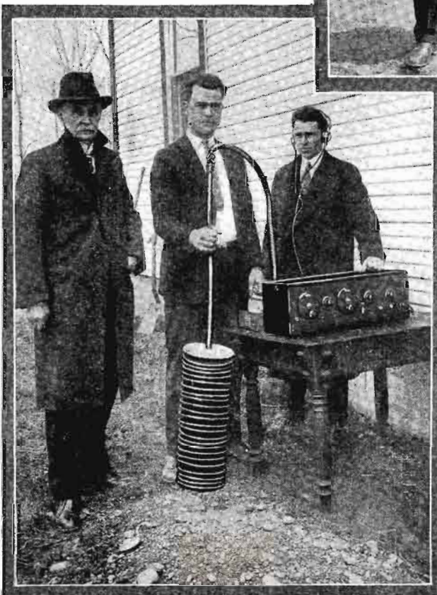
Above is shown Dr. Rogers, holding the household poker, by which satisfactory reception was obtained from amateur short-wave stations up to a thousand miles.
