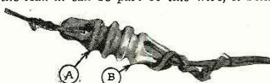
One year's accumulation of dirt and oxide on an aerial insulator. Note the contrast between section A and section B which has been cleaned.
