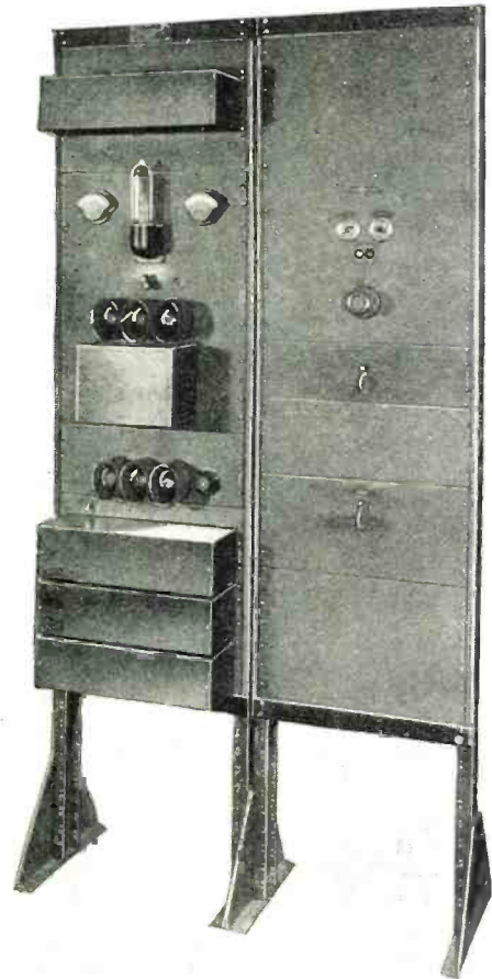
Fig. 4. A Carrier-Current Telephone panel for use in connection with high-voltage power-transmission lines.
