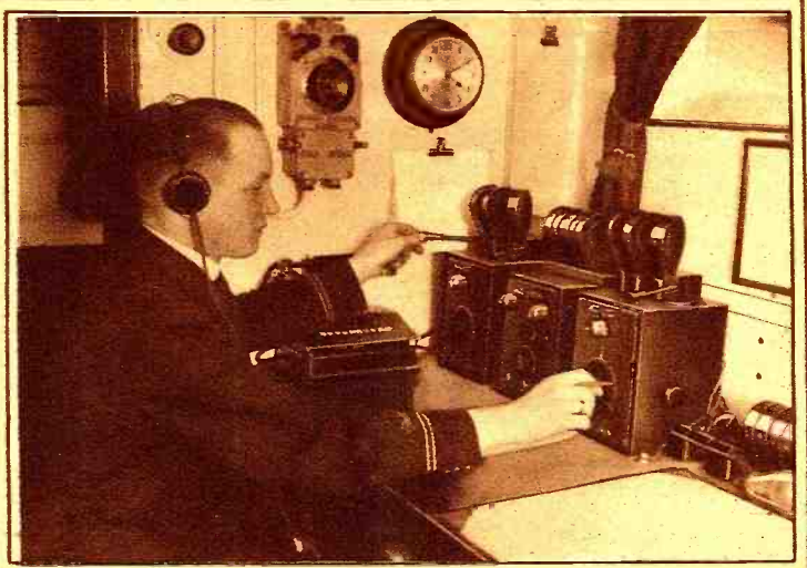
The short wave transmitter shown at the left will be used in the Greenland Expedition of the American Museum of Natural History. This transmitter has 250 watts power and is built to operate between the wavelengths of 13 and 45 meters. © Herbert Photos.
