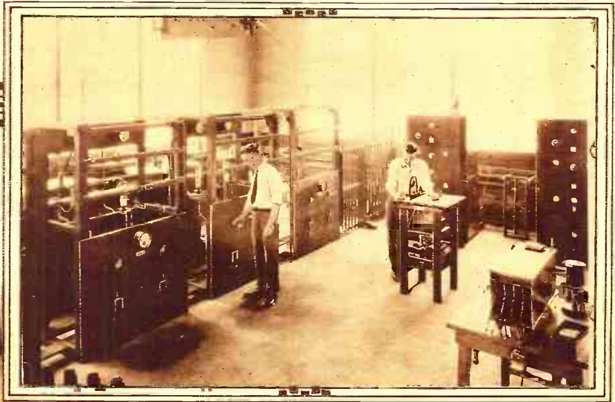
THE SUPERPOWER TUBES. These three units house the water-cooled tubes with their attendant step-up tubes and transformers. The two solid panels at the side are the terminal boards for the land lines that come from the studio in Schenectady.
