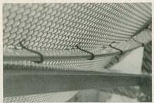
USE PLENTY of clips! In many designs, the mesh surface adheres to supportive under structure only when lashed down with clips. If you use too few clips, the system will not perform to specifications.
