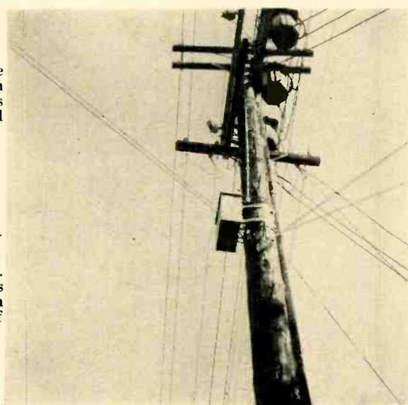
→ Two-set distribution outlet. Amplifier is mounted in weatherproof housing.
