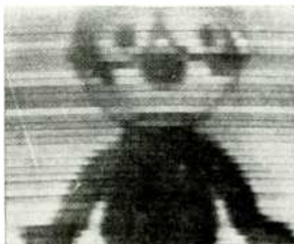
Felix the Cat was the "stand-in" when this 60-line image was made mechanically in tests at NBC's first experimental television station.
