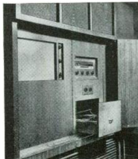
Fig. 5—Closed doors hide this installation.
