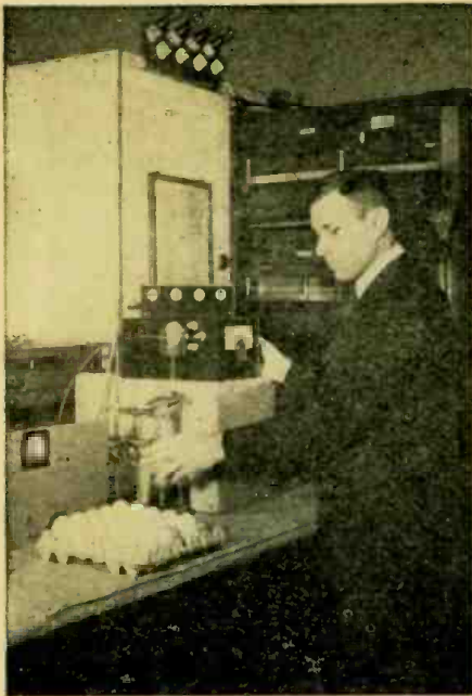
The inventor demonstrates the egg grader.
