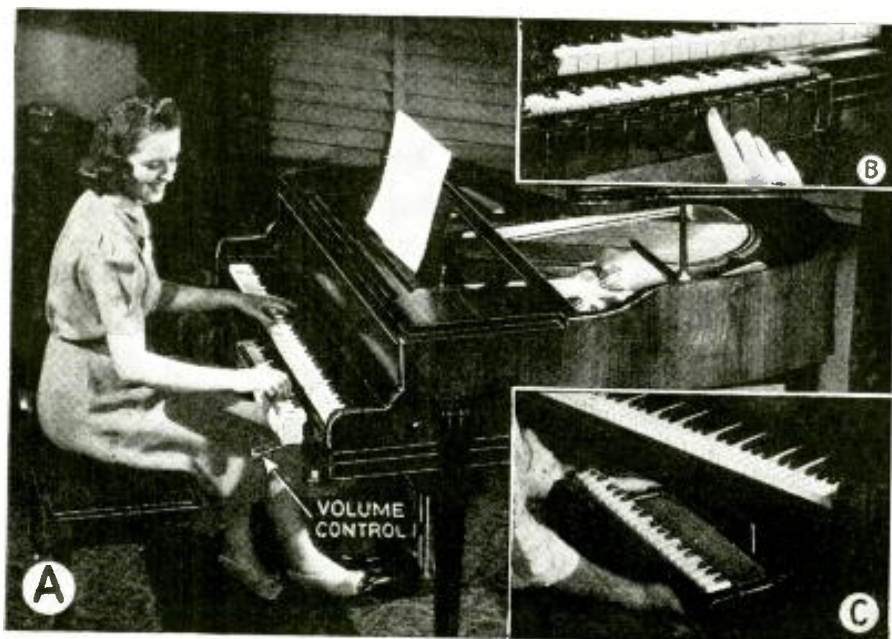
← The photos at left illustrate various elements of the Solovox. At A, the attachment in use on a grand piano, a set of 12 control tablets giving any piano an indefinite variety of tone colors that simulate the organ (Note individual volume control.); B, close-up of upper portion of the Solovox showing how the control tablet add-on device is fitted to produce a desired effect; C, the Solovox keyboard being attached to the piano keyboard by thumbscrews.
