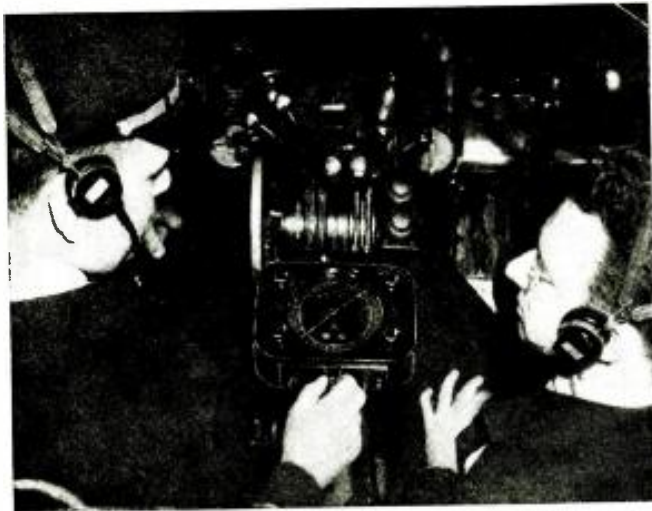
Left, modern installation of Sperry Automatic Direction Finder, in a Douglas Transport Plane. Special training is needed to service these instruments . . . no "slip-shod" mechanics wanted here!
