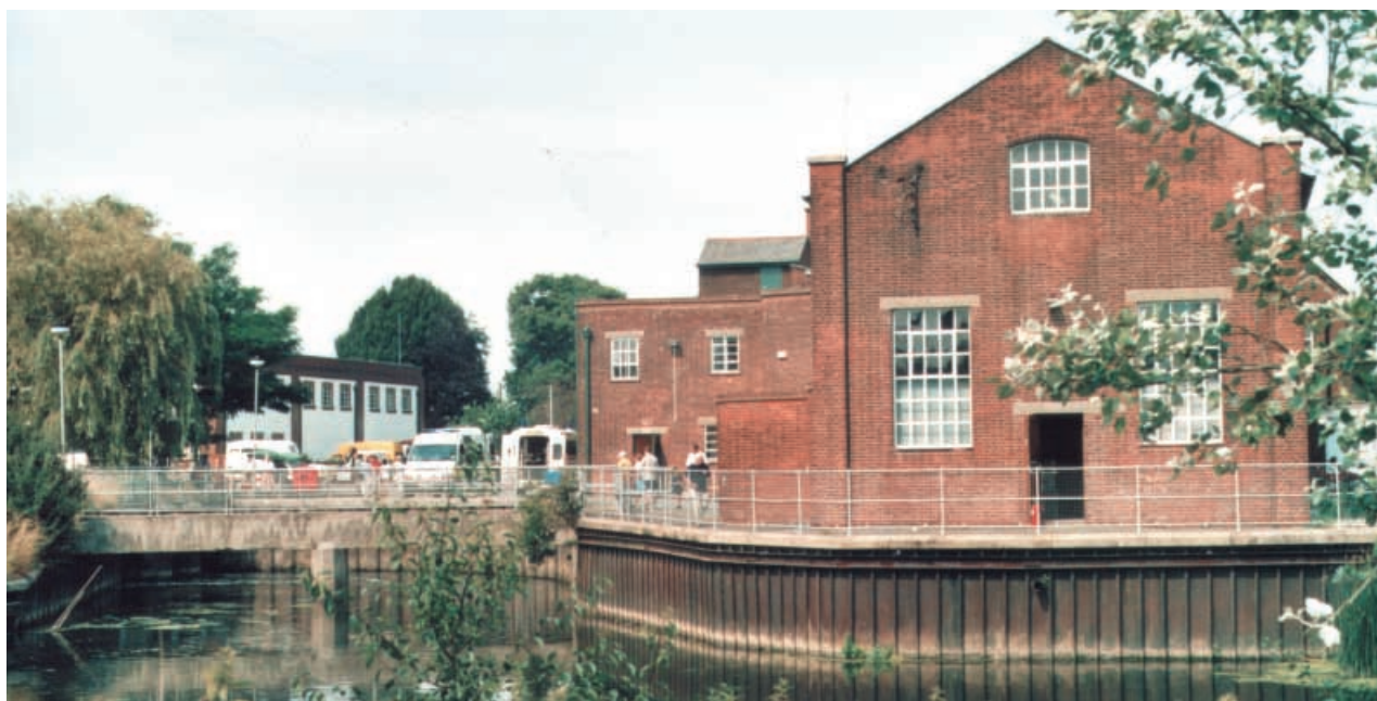
The Engine House, Sandford Mill
