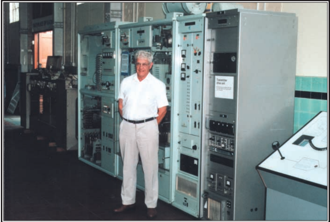
Geoff Lovegrove, G7KLV standing in front of the H1200 30kW transmitter. The large cylinder on the top of the cabinet is the low pass filter
