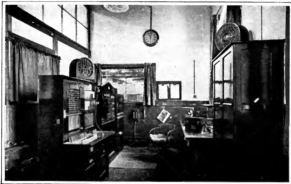
CONTROL ROOM OF 3 LO, MELBOURNE
