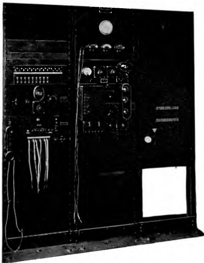
CONTROL EQUIPMENT OF THE PRAGUE, CZECHO-SLOVAKIA STATION
