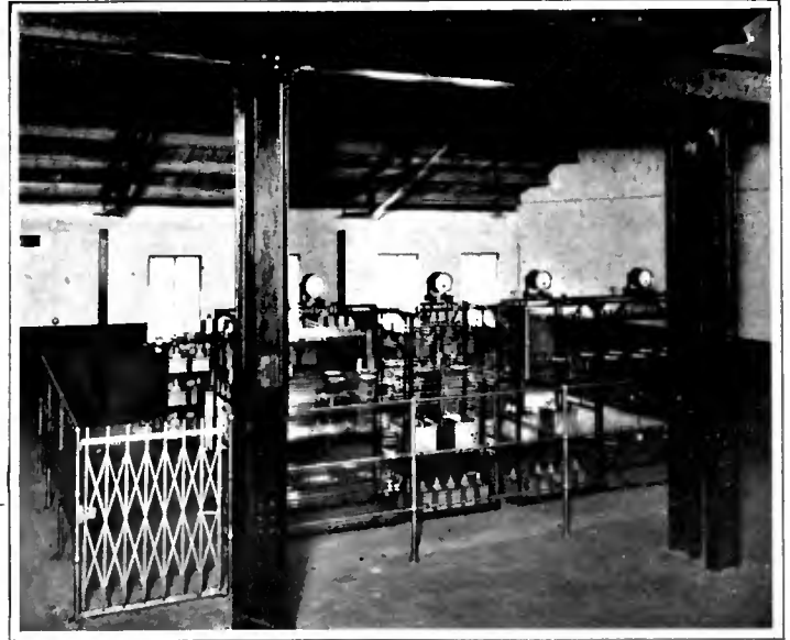
BEAM STATION EQUIPMENT
