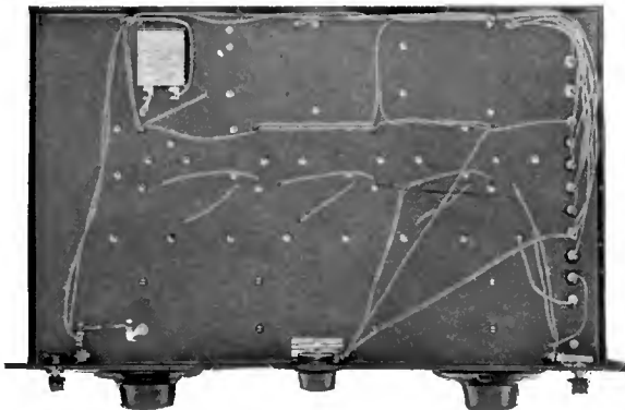
BENEATH THE SUB-BASE
