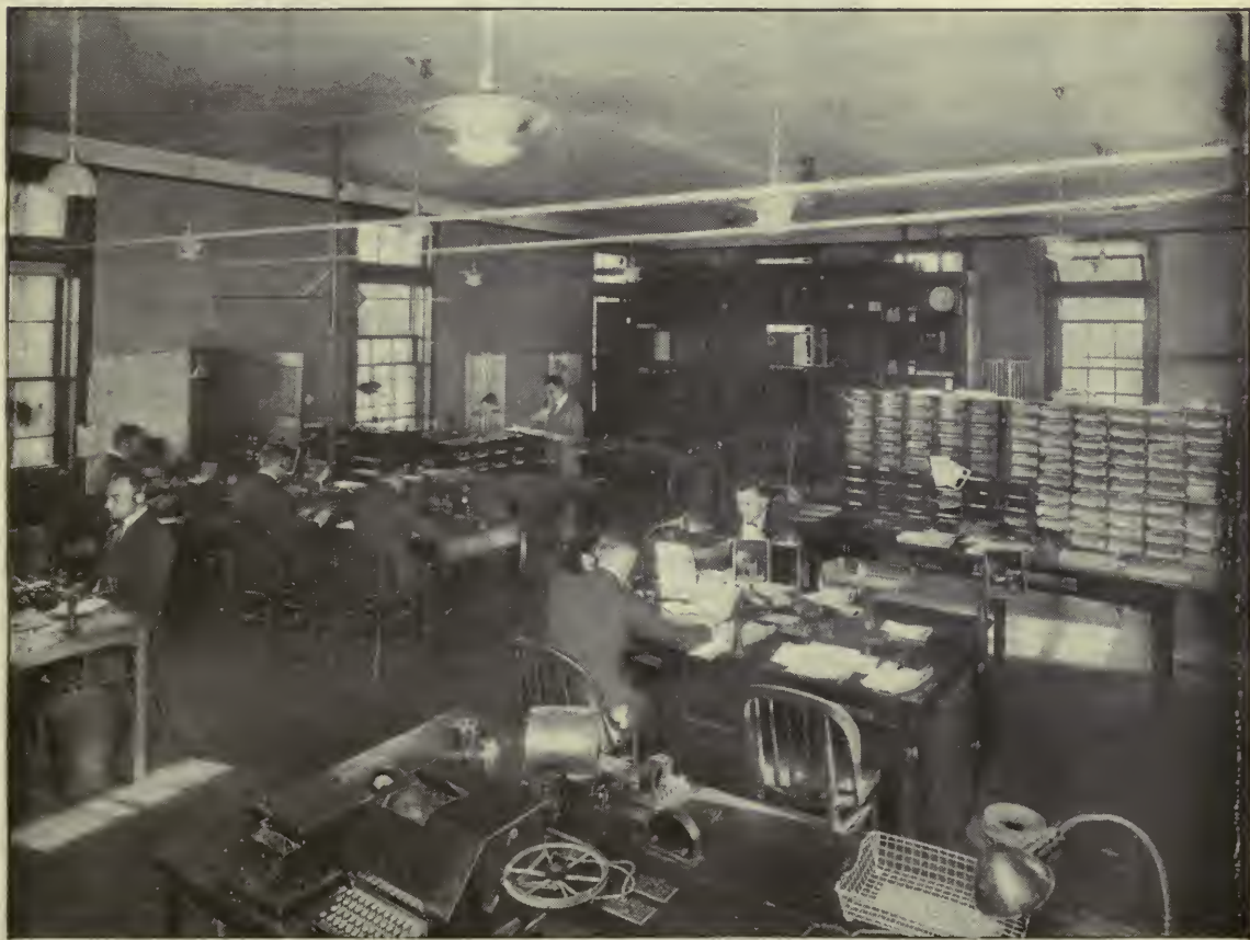
A VIEW OF THE CONTROL STATION AT BROAD STREET, NEW YORK CITY
