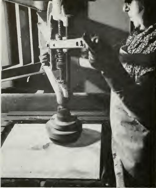
A copper-clad sheet of plastic, on which electronic circuits will be printed by photography, is highly polished before the light-sensitive emulsion is applied.
