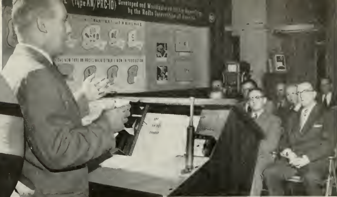
A Teleprompter user, reading his speech as it unrolls before him, is able to make his delivery sound extemporaneous. At left: An operator in the wings, working from an identical typewritten version of the text, adjusts the speed of the Teleprompter to the vocal speed of the speaker.
