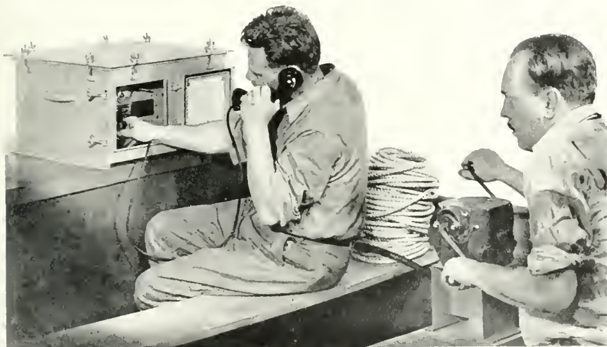
SPECIAL RADIO COMMUNICATION UNITS, DESIGNED BY ENGINEERS OF RADIOMARINE FOR LIFEBOATS, ARE PROTECTING LIVES OF THOUSANDS OF AMERICAN SEAMEN.
