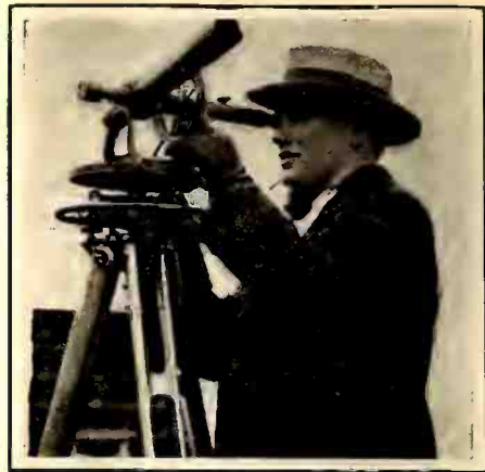
The weather man does use a telescope, but not to observe the moon. This shows James M. Brady, of the U. S. Weather Bureau at Washington, observing a pilot balloon with a theodolite. Twice a day, at Washington, and a number of other places, these small balloons are sent up and watched till they disappear from sight, to determine which way the air high overhead is moving
