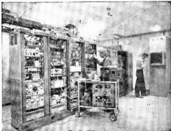
Final testing in progress at the New Plymouth terminal station of the New Zealand microwave telephone network (installed by STC). The four equipment cubicles on the left are the transmitter and receiver equipments for the "working" and "standby" radio channels. The supervisory VHF radio equipment is in the background.
