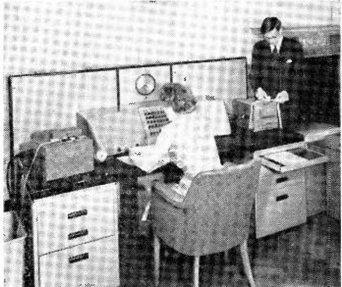
The Ferranti Sirius, a new transistorised desk-size electronic digital computer.
