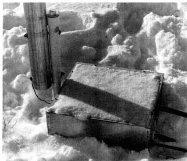
fig. 7. The remote control box should be located as close as possible to the base of the vertical.
