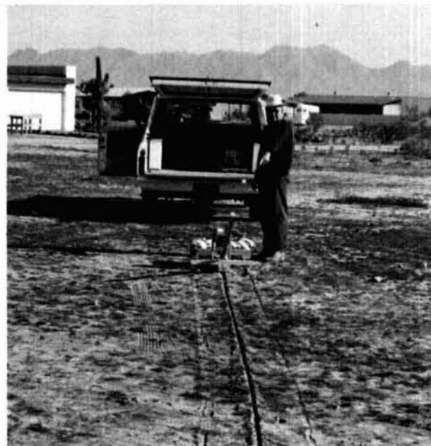
fig. 5. W7IR, shown here, guided plow while author drove 4 × 4 in low gear; plow can also be pulled by garden tractor or conventional auto.
