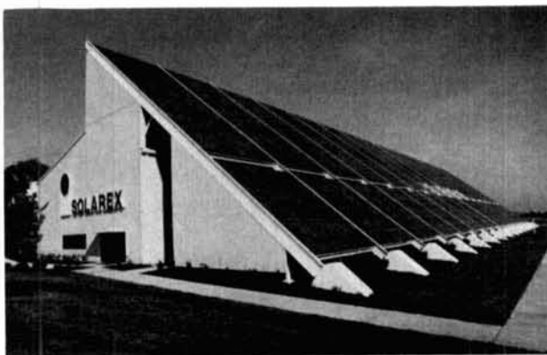
fig. 1. "Breeder concept" structure uses solar energy to provide power for production of solar cells.
