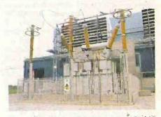
Four 400kV transformers connected to the outputs of the four generators.
