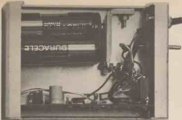
Top view with cover removed clearly showing the battery pack retaining bracket.
