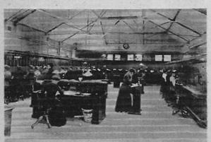
lines were routed. You picked up the receiver, turned a crank and the exchange answered by plugging one of a pair of plugs into your line.
