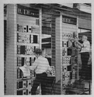
The first pulse code modulation tandem exchange (Post Office)
