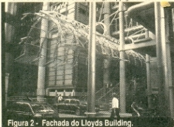
Figura 2 - Fachada do Lloyds Building.
