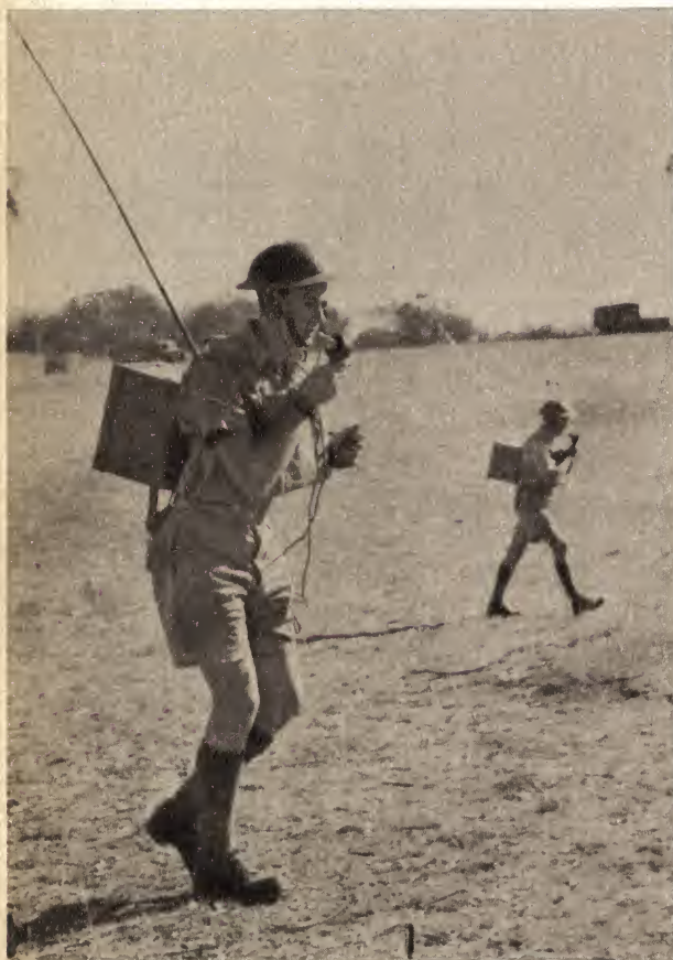
Back-pack radio telephones ("walkie-talkie") as used by British forces during World War II.
