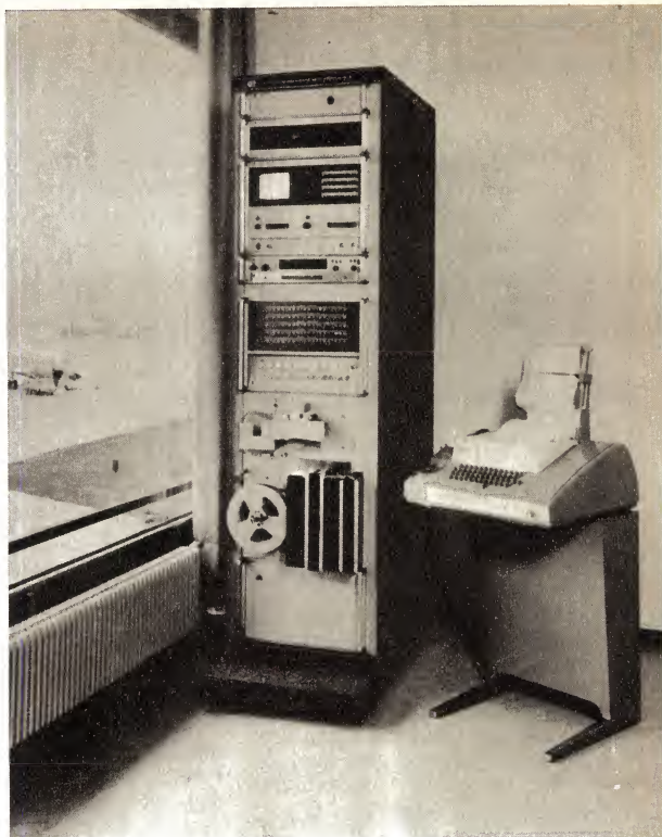
The central processor for an airport monitoring system. This can scan each noise monitoring terminal once each second, process the data obtained, and present the results in the optimal form for evaluation by relatively untrained personnel. It can be adapted to future regulations and noise evaluation methods simply by changing programs.
