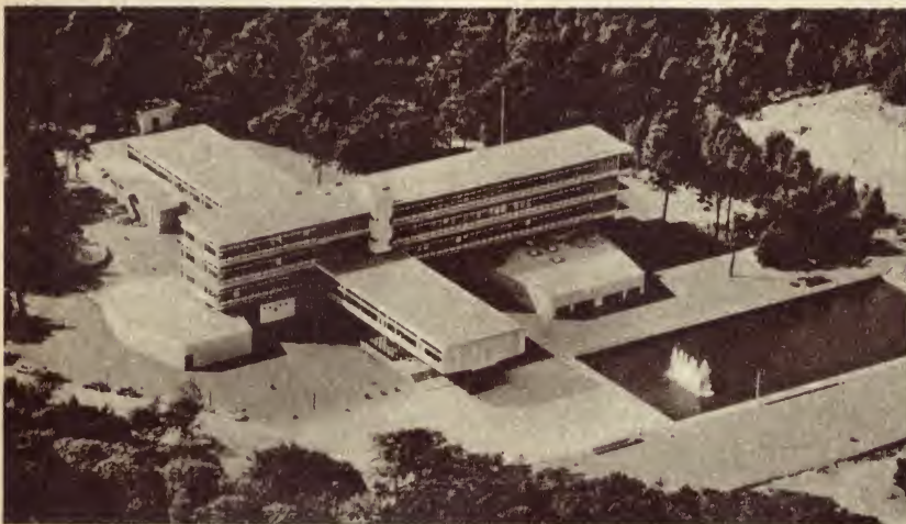
The magnificent modern building housing the studios of Hilversum Radio, in Holland.
